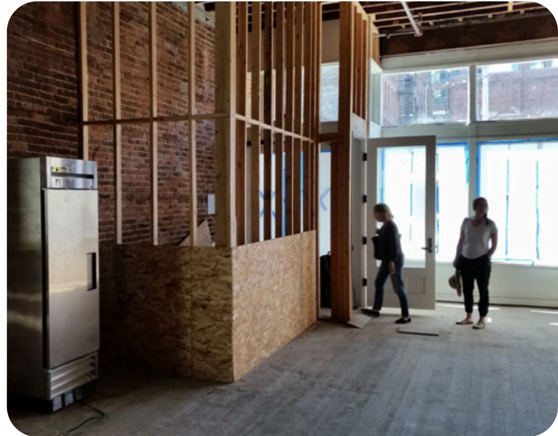
Elm Coffee Roaster, just beginning construction
